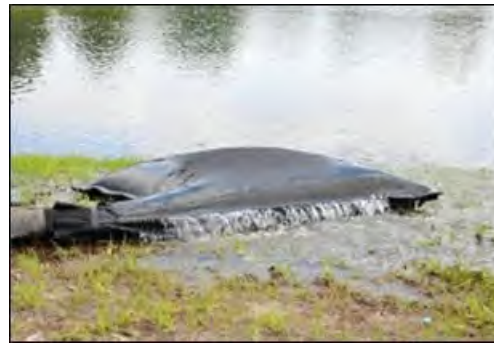
Plate 2-2 Silt Bag with water being pumped through
