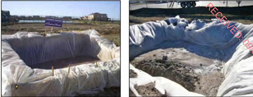
Plate 3-1 Typical concrete wash out areas
