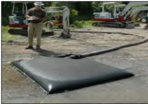
Plate 2-1 Silt Bag under inspection
