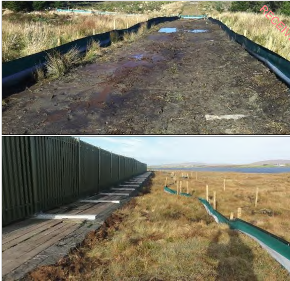
Plate 2-4 Typical Silt Fence Details
